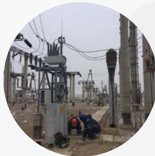
SUBSTATION CIRCUIT BREAKER
